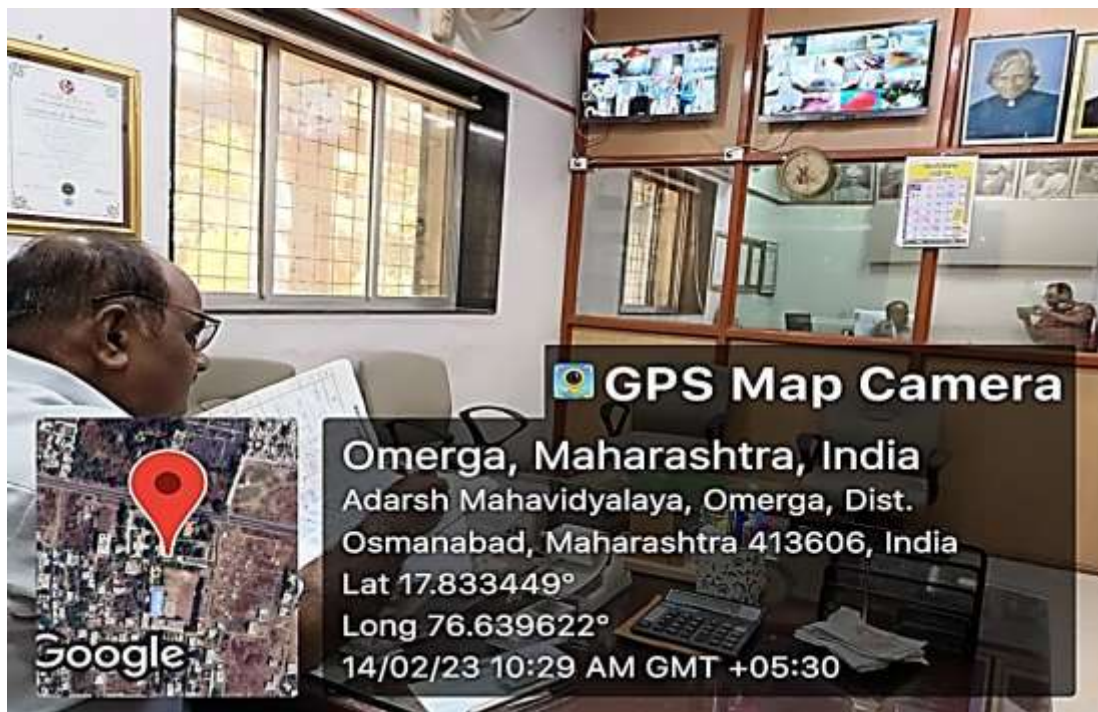
CCTV monitoring in Principal's Office
